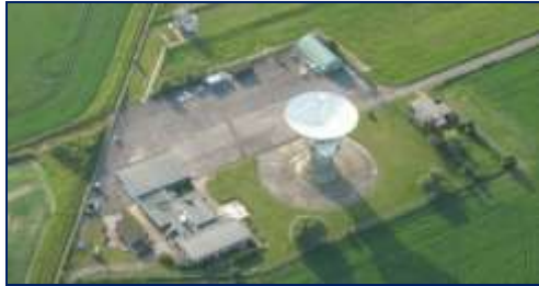
25m Dia. Antenna, Control Buildings and Support Labs
