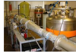
Pre-cooler frost control 2004
