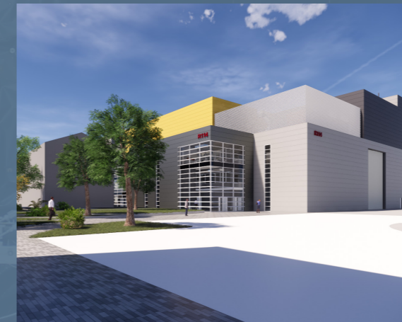
Artist's impression of the National Satellite Test Facility. Credit: STFC RAL Space/ Mace/ IBI
