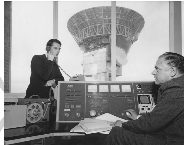
Chilbolton Observatory control room in 1967. Credit: STFC RAL Space
