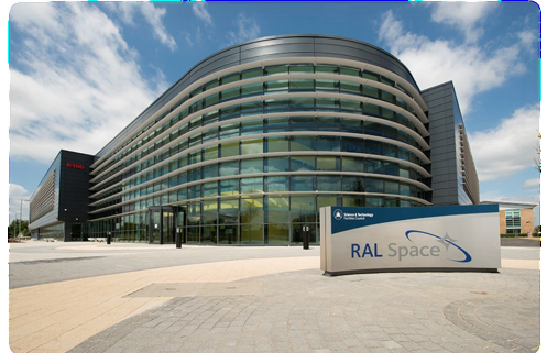
RAL Space Development and Integration Facility
